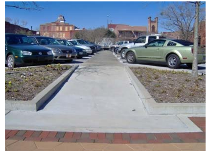
Figure 4-22. Pedestrian access was successfully incorporated into the parking lot design of this downtown lot in New Bern, NC.
