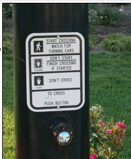
Figure 4-5. Examples of pedestrian-activated, signalized, mid-block crossings.
