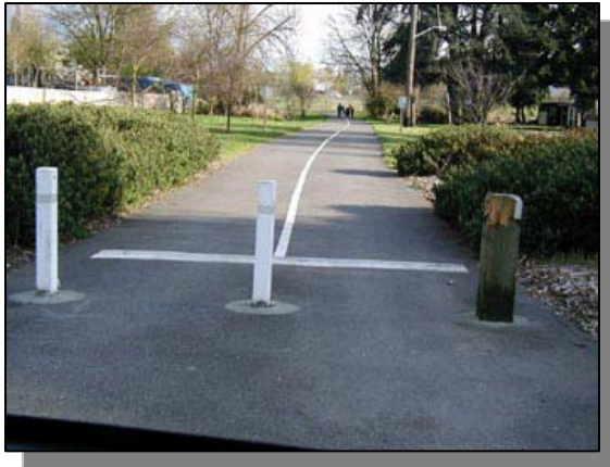
Figure 4-15. Typical greenway cross-section with bollard treatments at roadway crossing.
