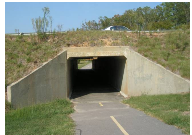
Figure 4-16. Pedestrian tunnels can be used to provide pedestrian connections under major roadways, active rail beds or other barriers. Effective lighting and visibility are essential to comfortable use by pedestrians and cyclists.
