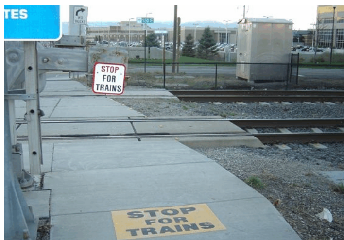
Figure 4-31. Pavement Marking and Counterweight-Mounted Warning Sign Source: FRA Compilation of Pedestrian Safety Devices in Use at Grade Crossings.
