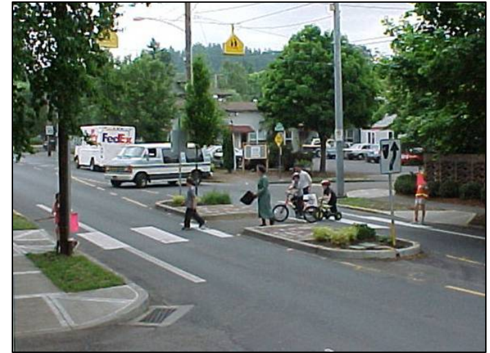
Figure 4-25. Example of a median refuge island in use. Source: www.pedbikeimages.com
