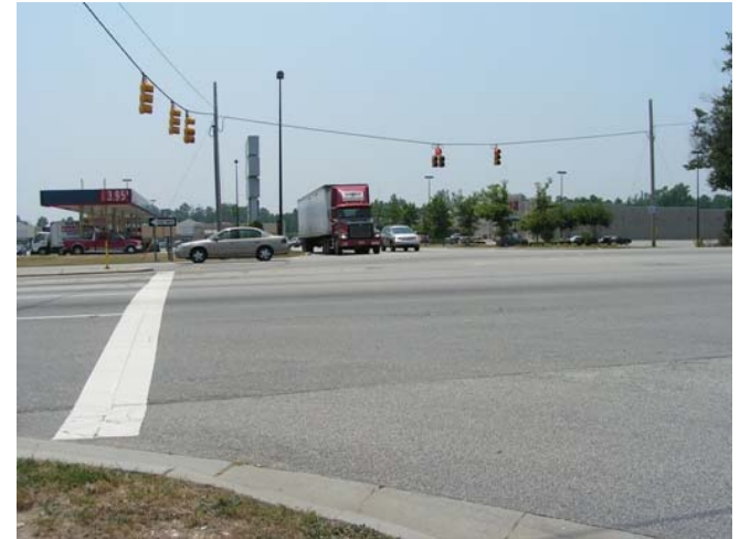
Figure 2-7. Wide crossing distances at intersections, such as on Cumberland Street at River’s Edge Center (above), were a top concern of Steering Committee members and other stakeholders. The use of crosswalks, median refuge islands and pedestrian signals at intersections with a designated “walk” phase could all help improve pedestrian access and safety along major thoroughfares throughout the City. Section 4 of the Pedestrian Plan recommends design standards for common intersection treatments.
